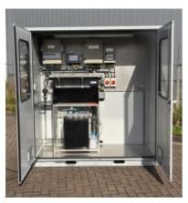
Interline's Early Warning System contains multiple online water quality measurement sensors for detecting natural, human-induced or deliberate contamination. If an incident is alarmed a water sample is automatically taken and a text message is immediately sent to your laboratory, which can then collect further samples for more detailed analysis.
